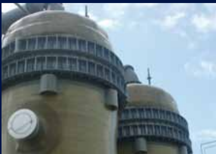
Two GRP reactors with PED approval (P = 8 barg, T = 80°C)
