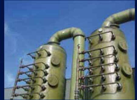
Two GRP scrubber to filter odors
