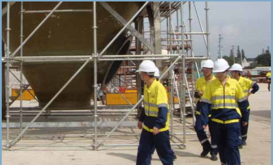
Assembly of a GRP separator for a chemical plant
