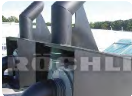
Polystone® G HD black Housing of a ventilation plant
