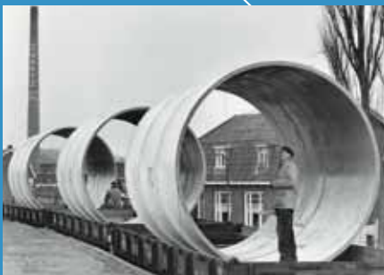
Transport of big diameter GRP cylinders to Germany in 1963
