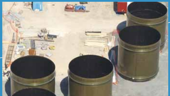
Stack liners (D = 10 meter) ready for installation
