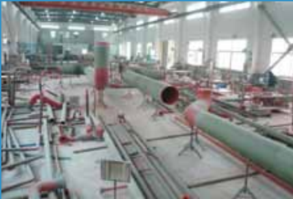
Preparation of dual laminate spools for a project in China
