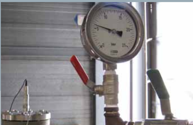
Hydrostatic test of a vessel with PED approval
