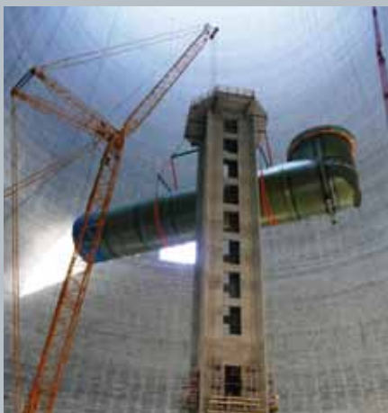
Lifting of a 10 meter diameter duct in a cooling water tower
