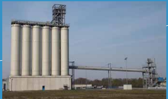
GRP silos (6 x 500 m3 D = 5000 mm)
