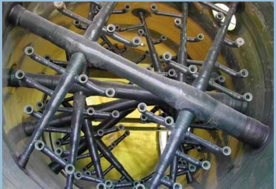
GRP spray header with a anti abbrasive protection layer on the top
