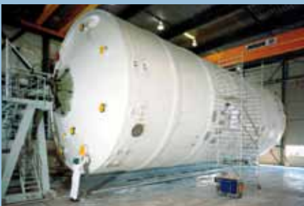
The production of a 1000 m 3 , 9.5 meter tank in one of our production facilities
