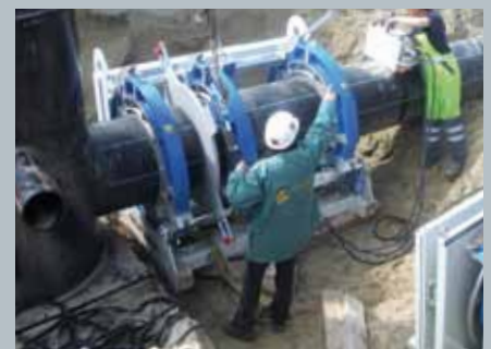
Installation of a thermoplastic (PE) pipe
