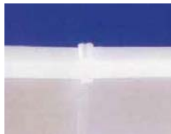
溶着接合部 Photograph of butt Fusion joint
